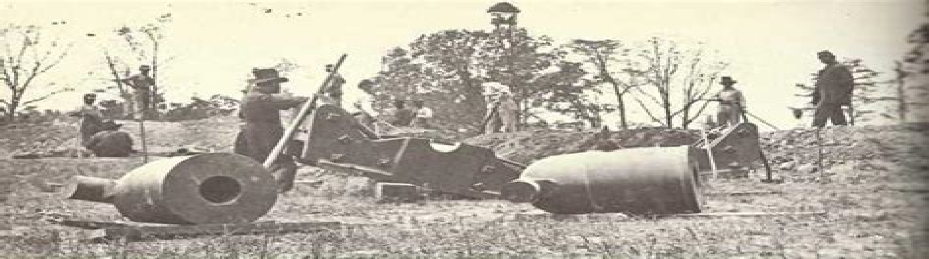
FIGURE: III-8 IDENTIFICATION: Mortar, Seacoast, 10-Inch, Model 1841-44, Iron. REMARKS: Mortars being emplaced at Butler's Cross Nest, Dutch Gap. Note clevis and bolt attached to mortar cars. COMMON NAME: 10-Inch Seacoast Mortar, Model 1841-44.
