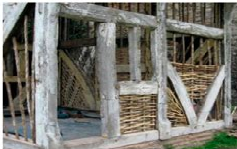
Figure 6. Wattle and Daub Infill Panels
