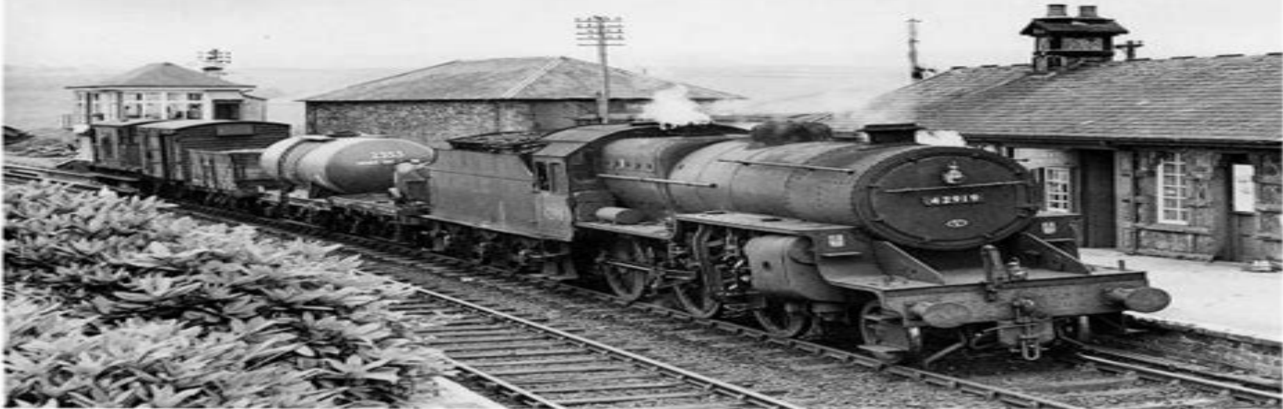
CREETOWN (SPITTAL LENNIES): 'Crab' 2-6-0 No 42919 pauses at Creetown station with a down pick-up freight on 15 July 1963. The loco is pulling forward to take water before heading for Stranraer. No 42919 was a Dumfries (68B) loco, spending many years at that shed. Michael Mensing
